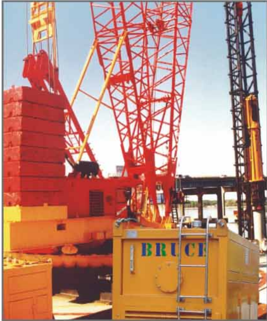
BRUCE SGH-3013 working at bridge foundation site at Panama City, Florida, USA driving concrete pile (O.D 60" x I.D 45" x 120 feet long)
