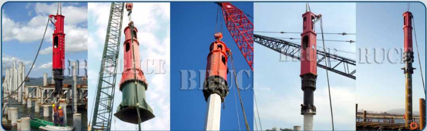
Hammers working with crane suspended type.
