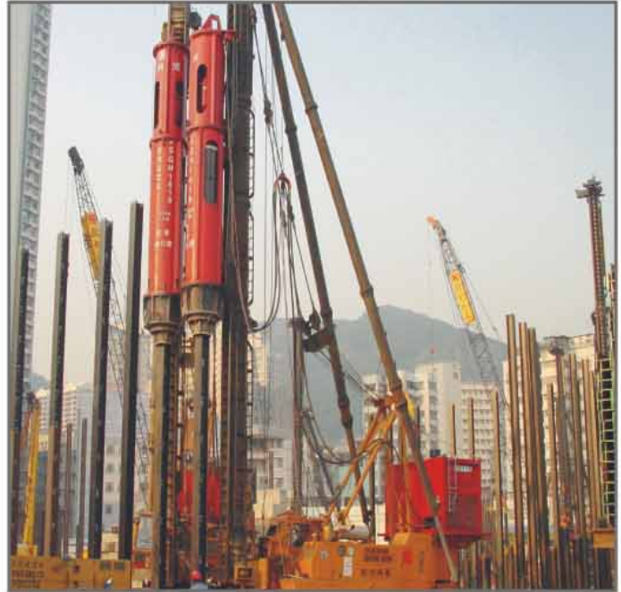
BRUCE SGH-1618 & 1619 at Hong Kong driving H-beam piles (305mmx 305mm, 223kg/m, 48m long)
